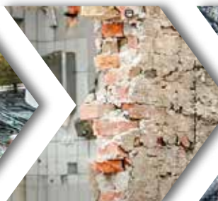
Concrete and mixed demolition material
