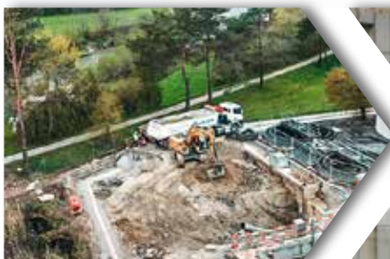
Excavated material and demolition debris
