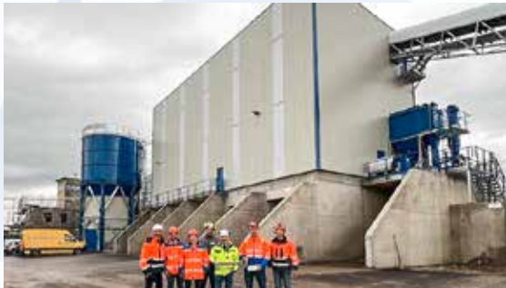
BRT Baustoff Recycling AG, Weinfelden Wet mechanical processing system
