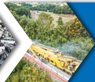
Excavation de rails
