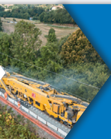
Excavation de rails
